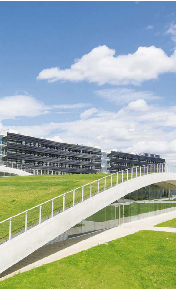
↑ Example of extensive green roof. Campus, Research Center, Marne La Vallée, France. Pic source: Archdaily
